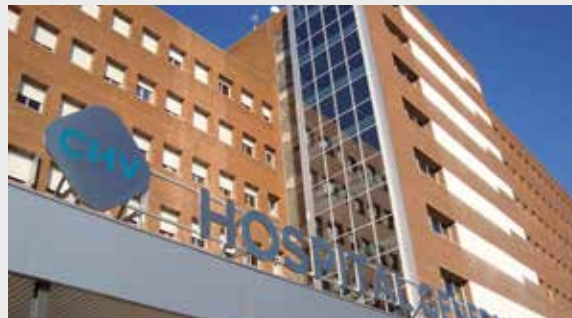
Hospital General de Vic
