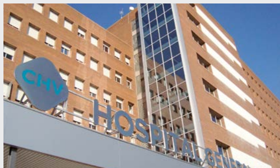
Hospital General de Vic
